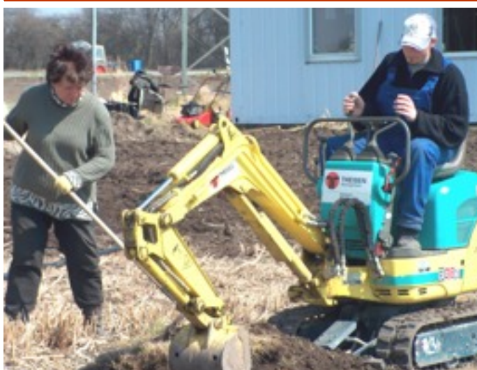
2. Digging trench for water-pipe
