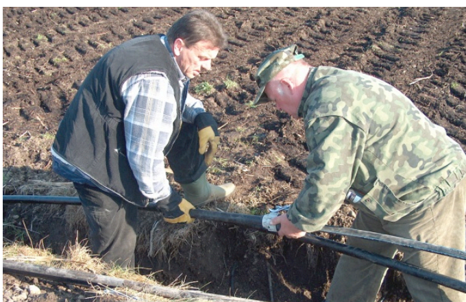
4. Connecting water-pipes
