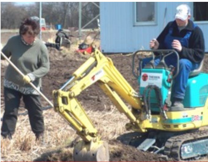
2. Digging trench for water-pipe
